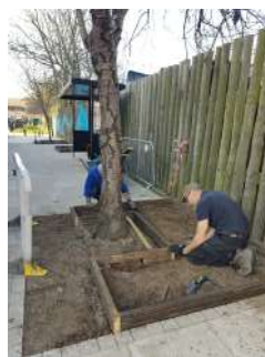
Retaining edges added
