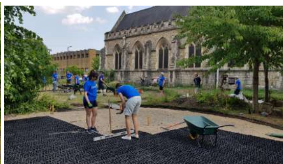
Plastic gravel grid made from recycled plastic in UK
